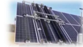
Robotised module cleaning
